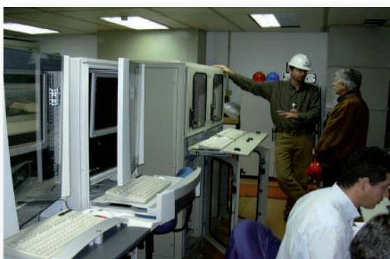
Control room of the ITaipu Dam
